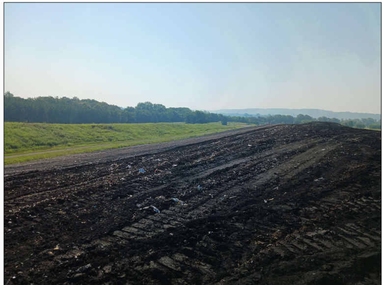
Photo No. 2 Looking south at the eastern slope of Area 5.
